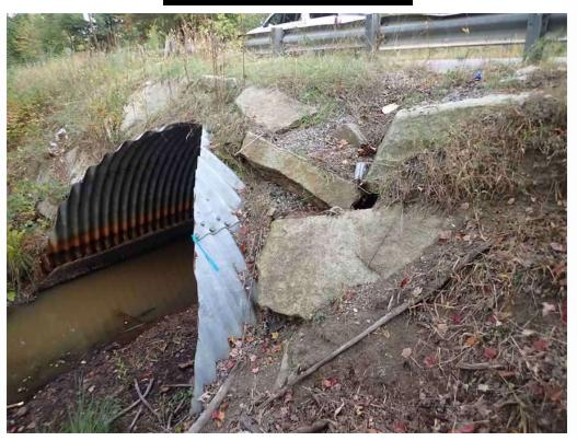
Photo 3: Settled stones and voids in the top east end of the south embankment.
