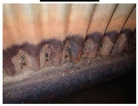
Photo 1: Typical laminar rust and section loss to the bottom 8" of the corrugated arch (east side shown).
