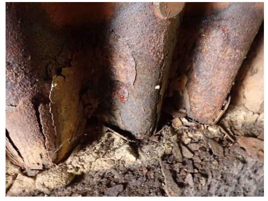
Photo 2: Typical laminar rust and section loss to the bottom 8" of the corrugated arch (east side shown).
