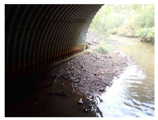
Photo 8: Aggradation at the southeast corner of the culvert.
