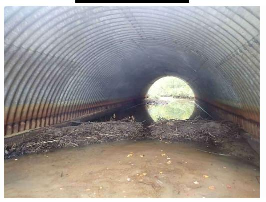
Photo 7: Debris pile near the north end of the culvert.
