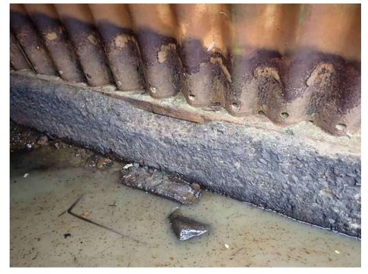
Photo 6: Spall to the top of the west abutment / footing near the north end.
