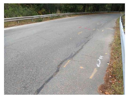
Photo 4: Longitudinal cracking to the eastbound lane of the wearing surface.
