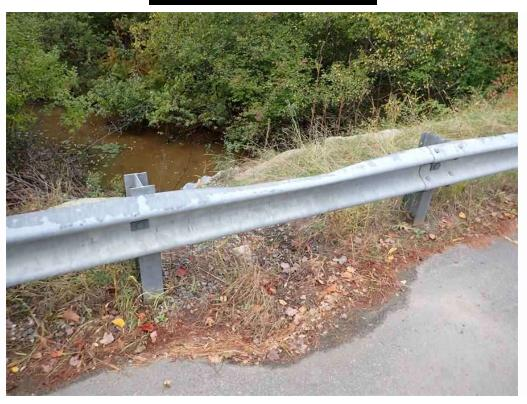
Photo 5: Damage to the top of the south railing near the east end.
