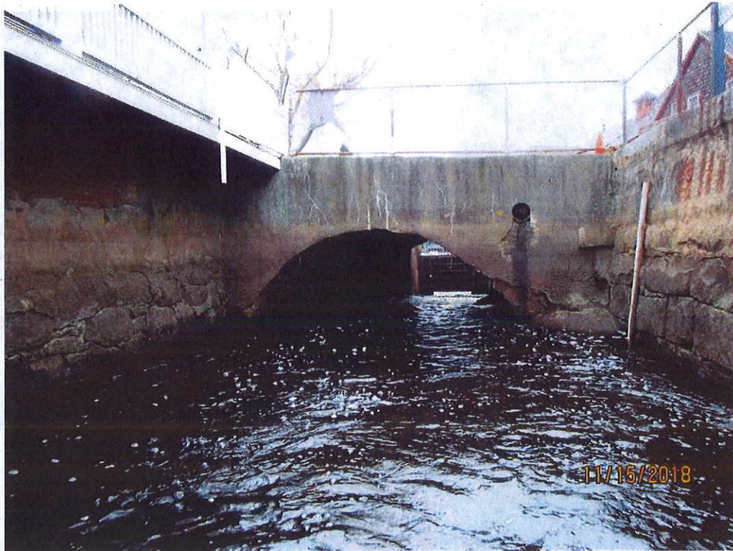
Photo 1: General - North elevation.
