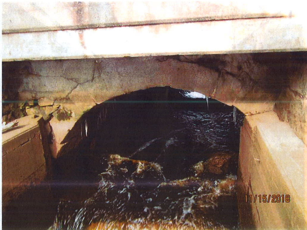
Photo 2: General - South elevation.
