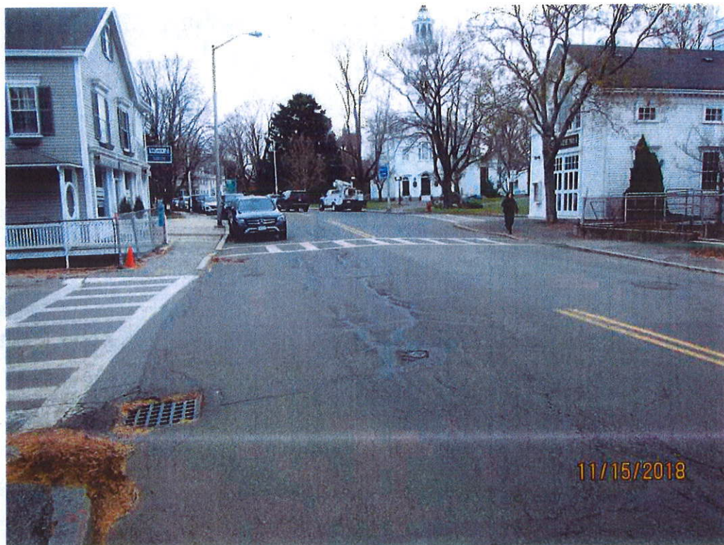
Photo 6: General - West approach, looking east.
