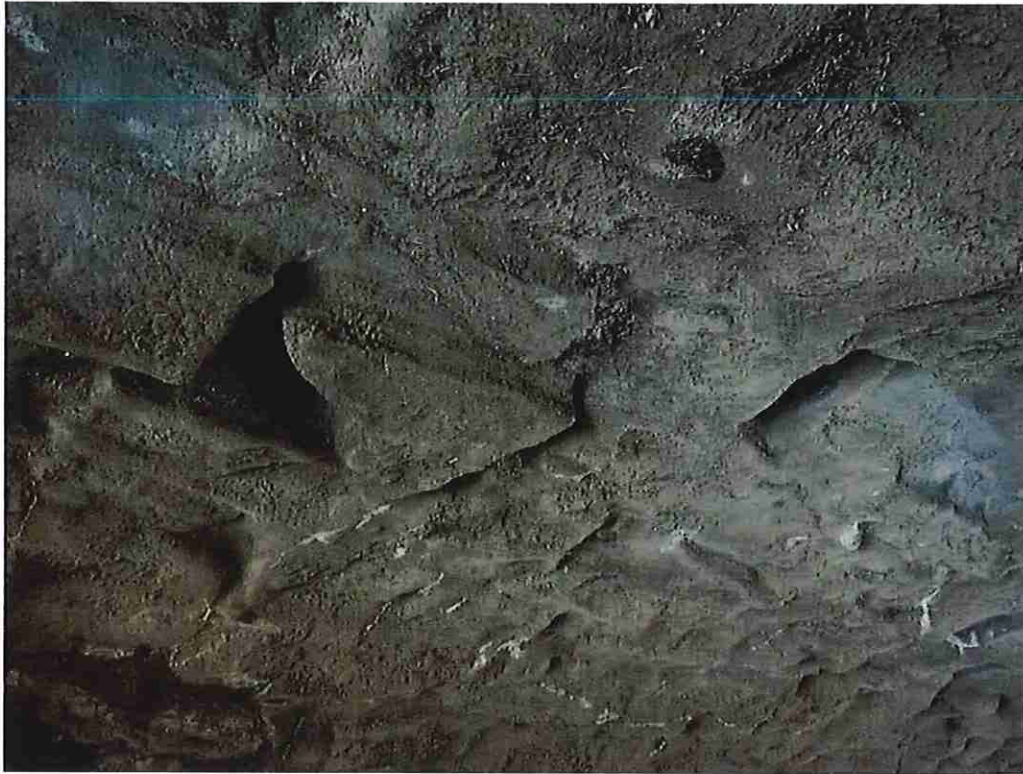
Photo 5: Triangular shaped void in the keystone area at 14' in from the north fascia.
