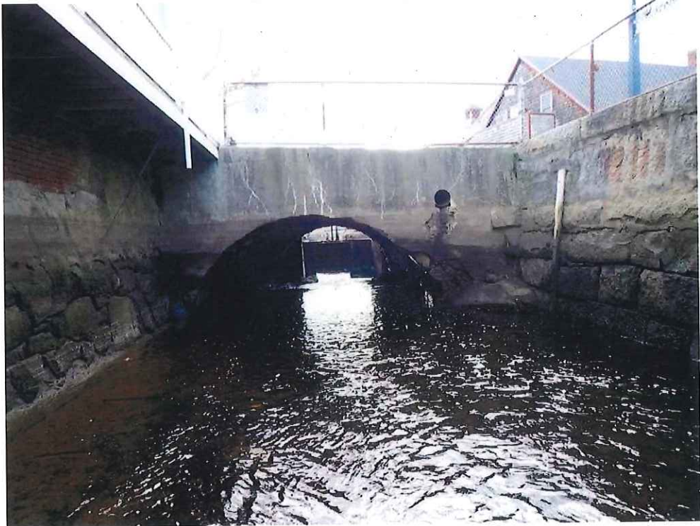
Photo 1: General - North Elevation.
