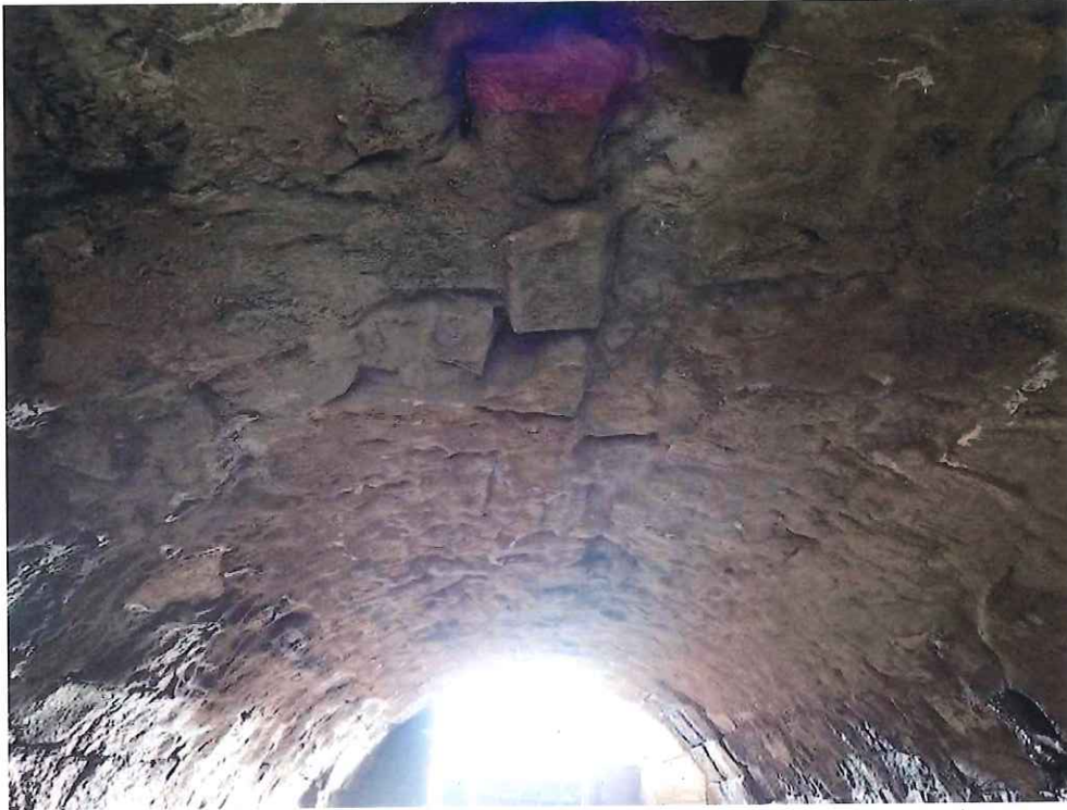
Photo 7: General - Typical underside, looking south.
