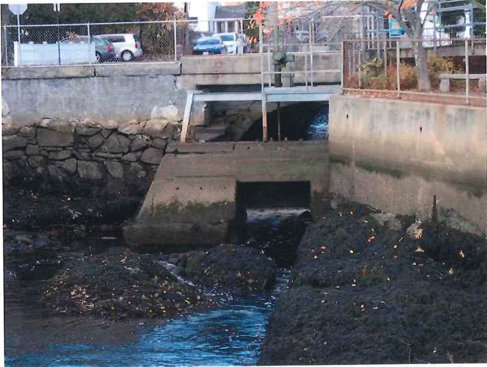
Photo 2: General - South Elevation (Bridge 8AM partially hidden beyond tide gate).
