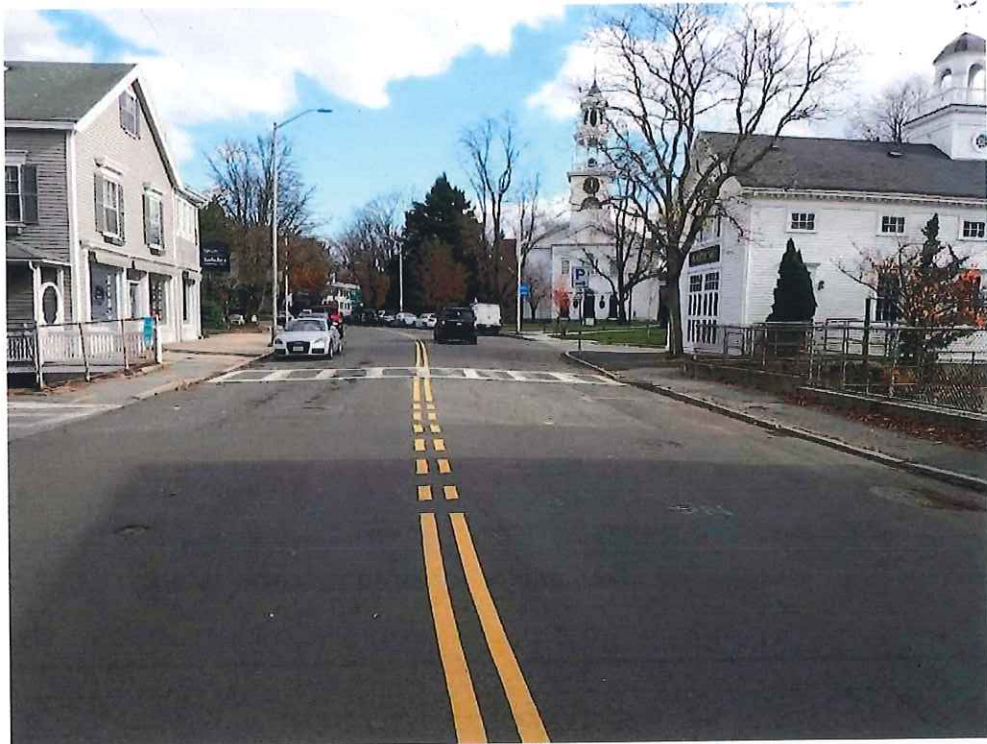
Photo 6: General - West approach, looking east.
