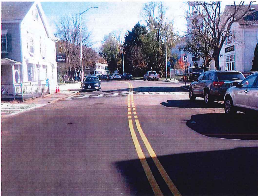
Photo 6: General - West approach, looking east.
