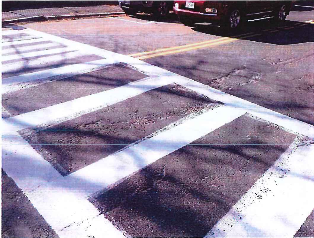
Photo 7: Wearing Surface- Westbound Lane: Heavy wear full length x 18" wide x 1/2" deep with scattered cracking.
