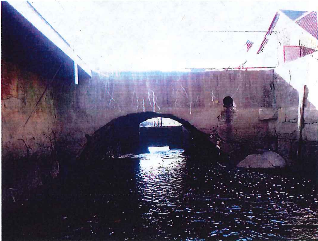
Photo 1: General - North Elevation
