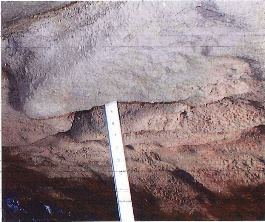
Photo 3: 14'-0" From North Fascia: 12" long x 8" wide x 6" deep void; stones surrounding void settled up to 6"
