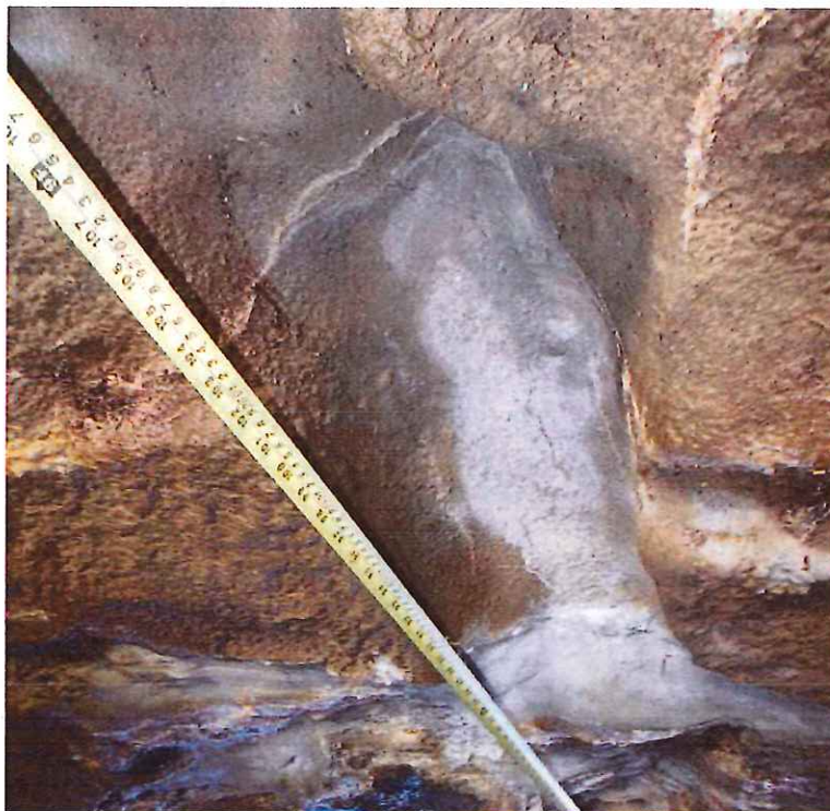
Photo 2: 7'-0" From North Fascia: 24" long x 9" wide x 5" deep void
