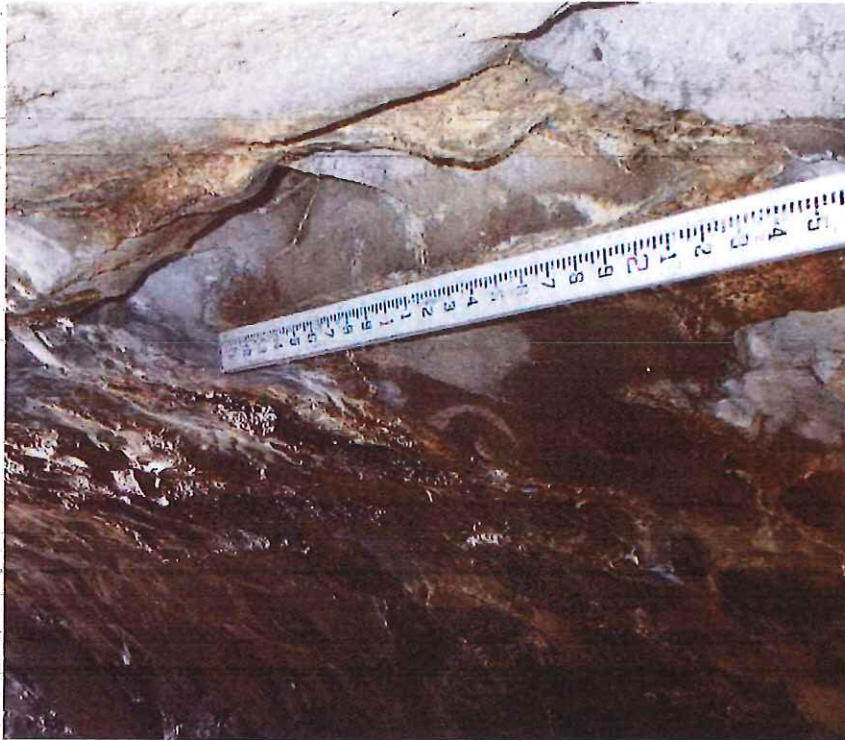
Photo 1: 2'-6" From North Fascia: 24" long x 9" wide x 6" deep void
