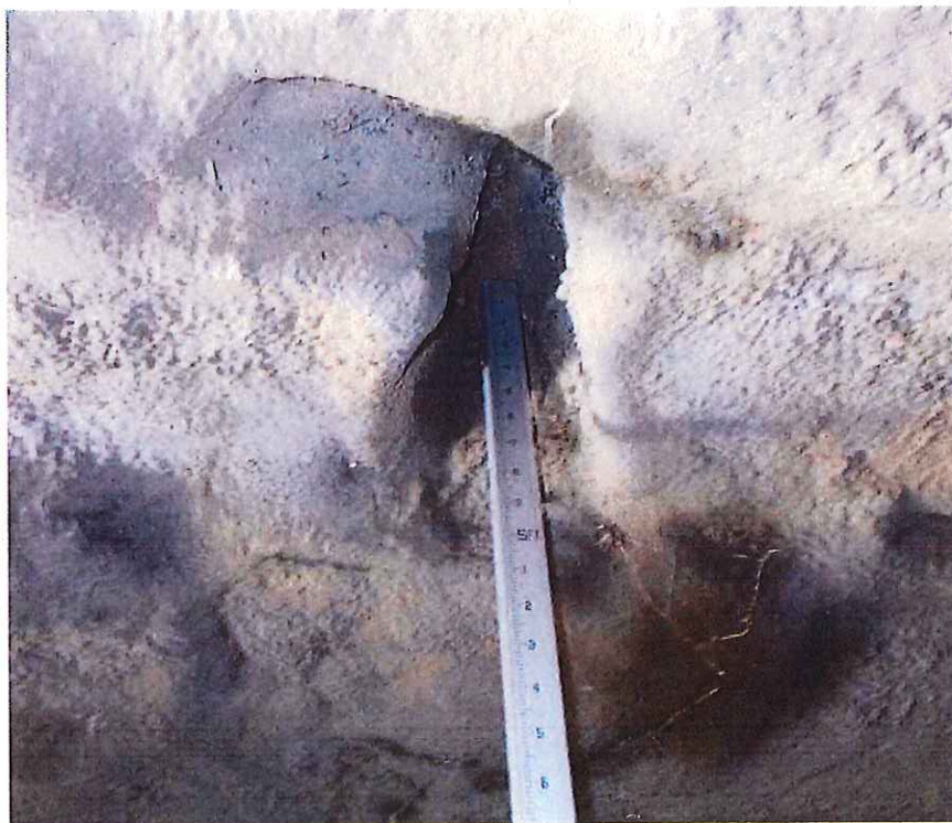
Photo 4: 17'-0" From North Fascia: 6" long x 12" wide x 9" deep void
