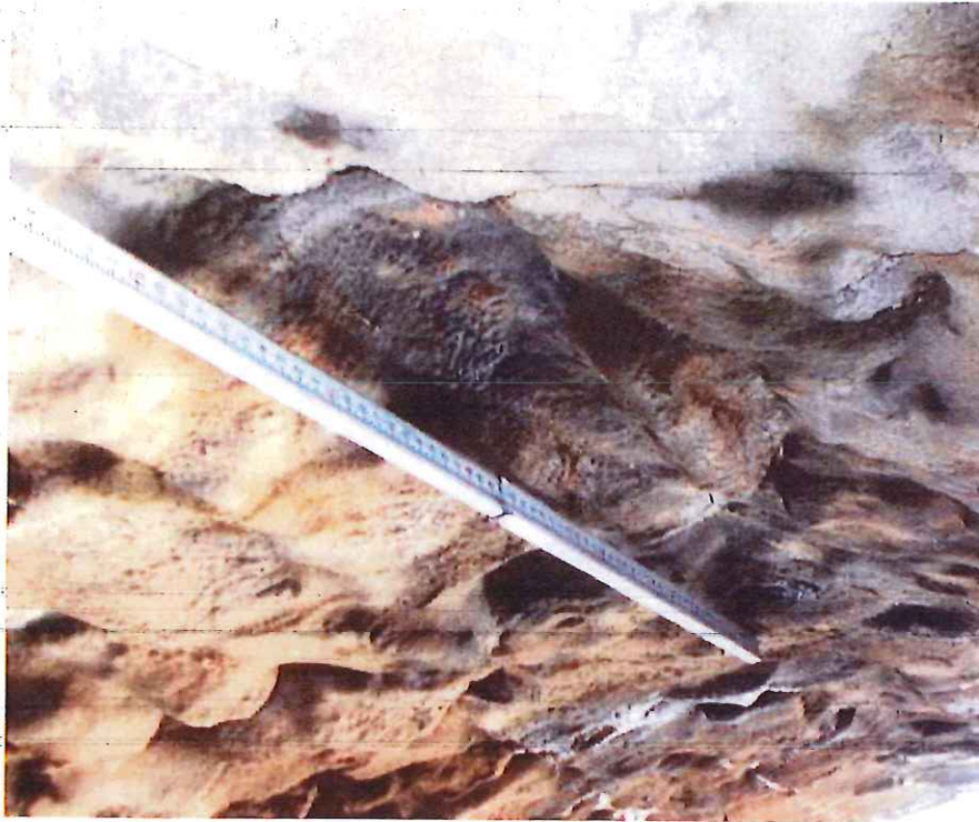
Photo 5: 22'-0" From North Fascia: 5' long x 12" wide x 6" deep void
