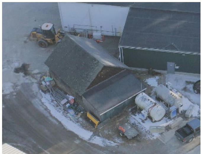
Honey Shed (west/rear side) (fuel island lower right)
