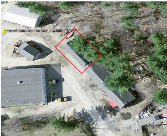
Historic Aerial Image – Former Storage Building
