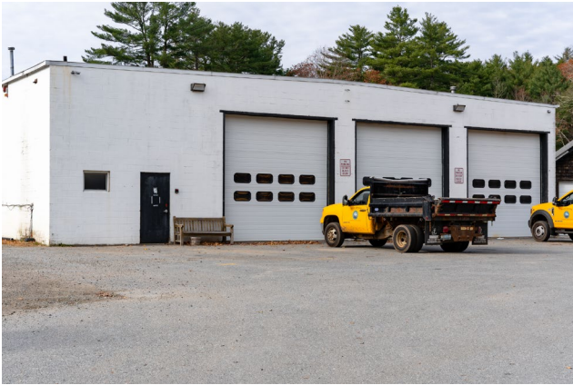
Maintenance Garage – Front (east)
