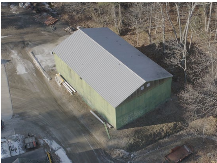
Salt Shed (east side)
