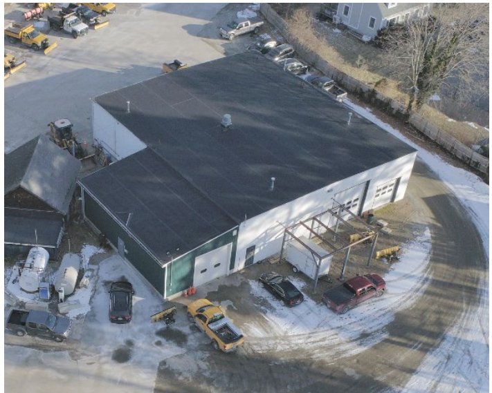
Maintenance Garage – Rear (west)
