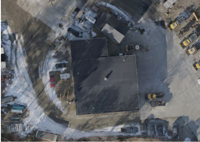
Maintenance Garage – Aerial View
