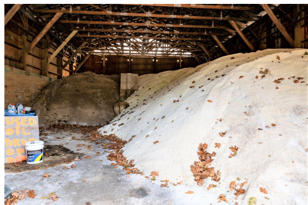
Salt Shed (interior)
