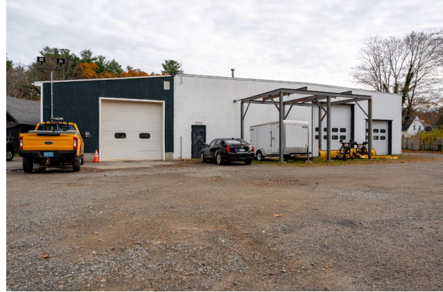
Maintenance Garage – Rear (west)
