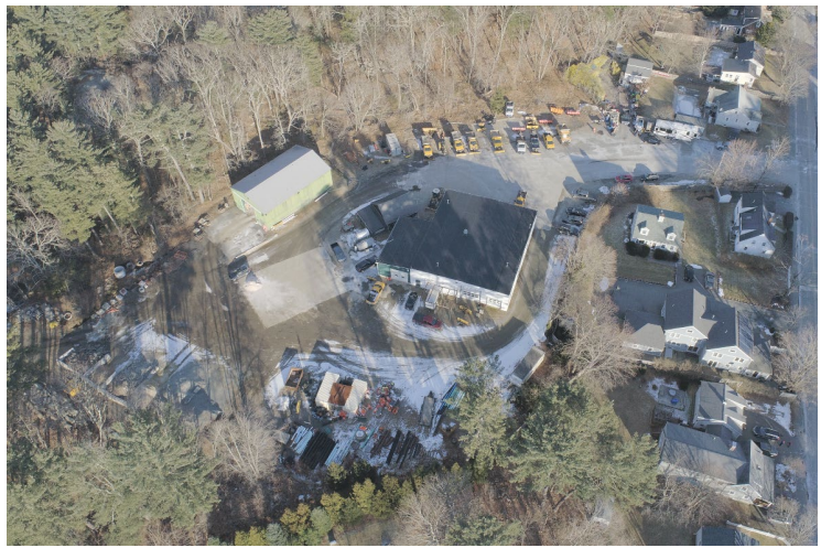
Aerial View – Looking East
