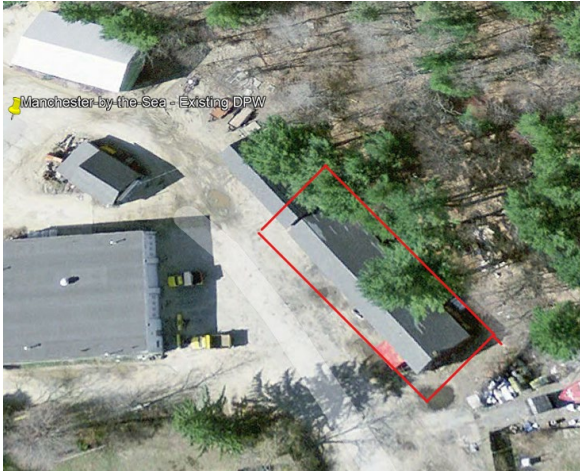
Historic Aerial Image – Former Storage Building
