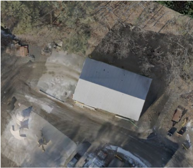
Salt Shed – Aerial View
