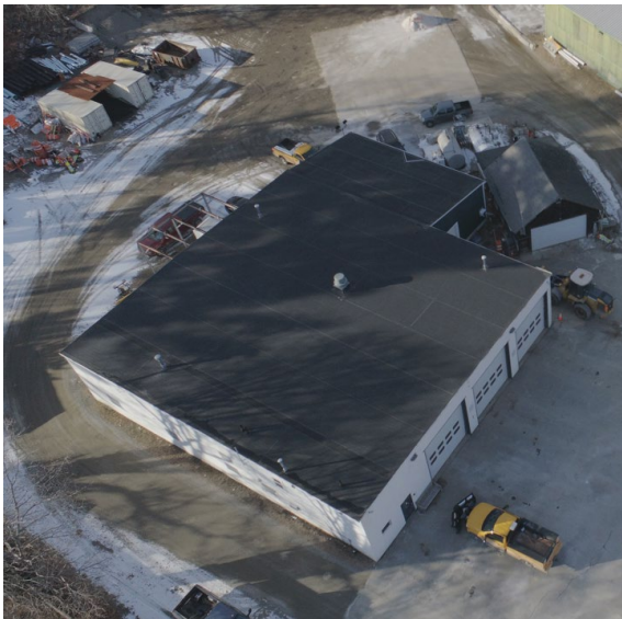
Maintenance Garage – Front (east)
