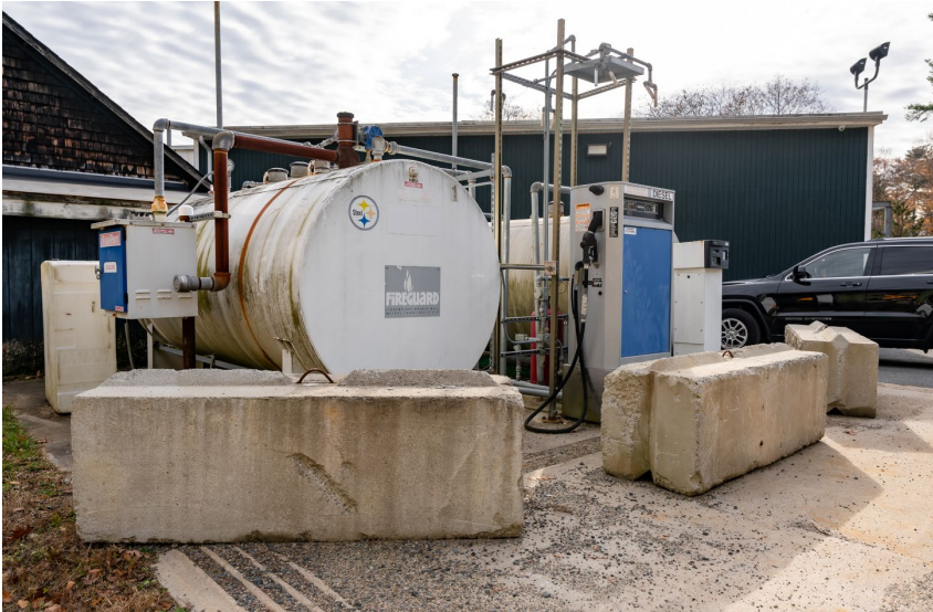
Fuel Island (looking south)
