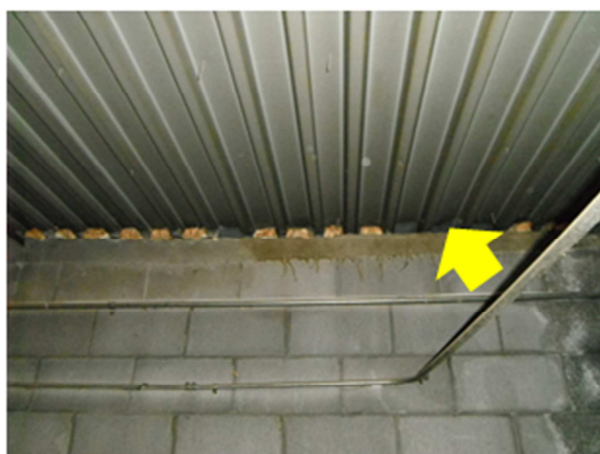
Roof-Wall Intersection Air Sealing – gaps between the roof deck and structure wall framing due to trusses at the roof-wall intersection are pathways for unwanted infiltration/exfiltration; the foam material has completely deteriorated and does not provide a tight seal.
