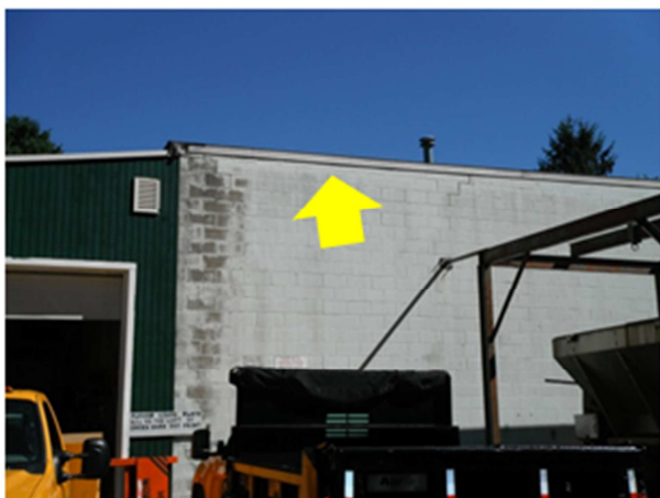
Roof-Wall Intersection Air Sealing – the exterior flashing and finishes at the roof-wall intersection are not constructed to stop air leakage.
