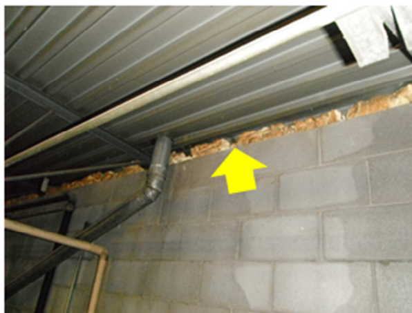
Roof-Wall Intersection Air Sealing – gaps between the roof deck and structure wall framing due to trusses at the roof-wall intersection are pathways for unwanted infiltration/exfiltration; the foam material has completely deteriorated and does not provide a tight seal.
