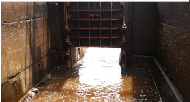
Photo 3: View of the tide gate from inside culvert
