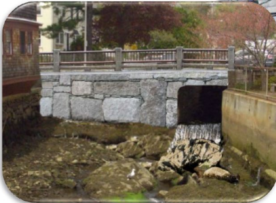
Photo rendering of tide gate removed, new culvert, new granite wall and guard rail
