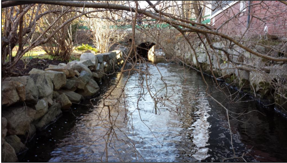
Outlet of School Street Culvert
