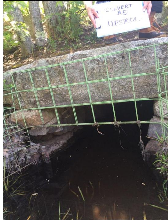
Inlet of one of Old School Street Culverts
