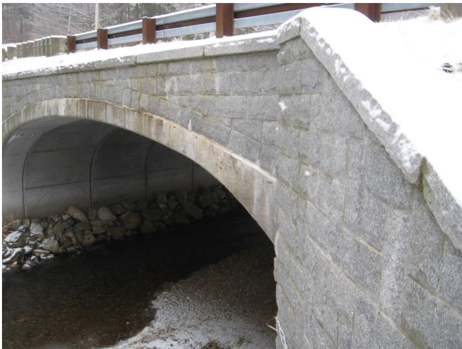
Figure 3 - Sample Stacked Stone Façade (Granite)
