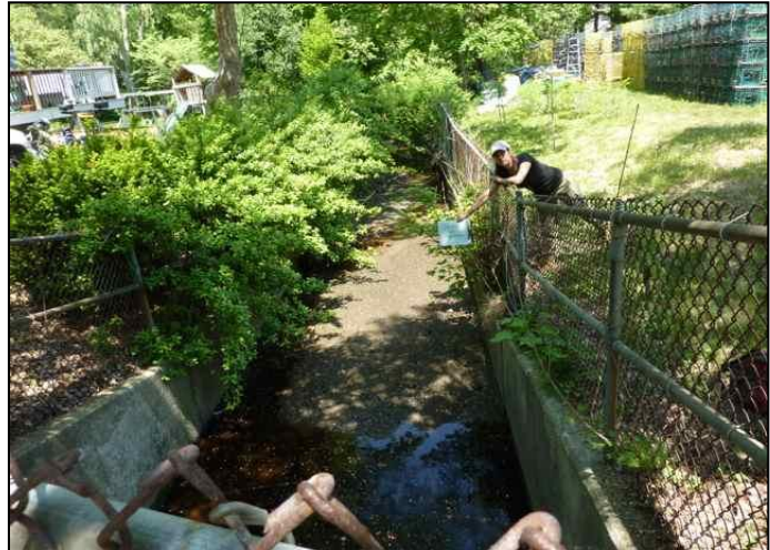
Causeway Brook downstream of Summer Street, showing the narrow channelized streambed
