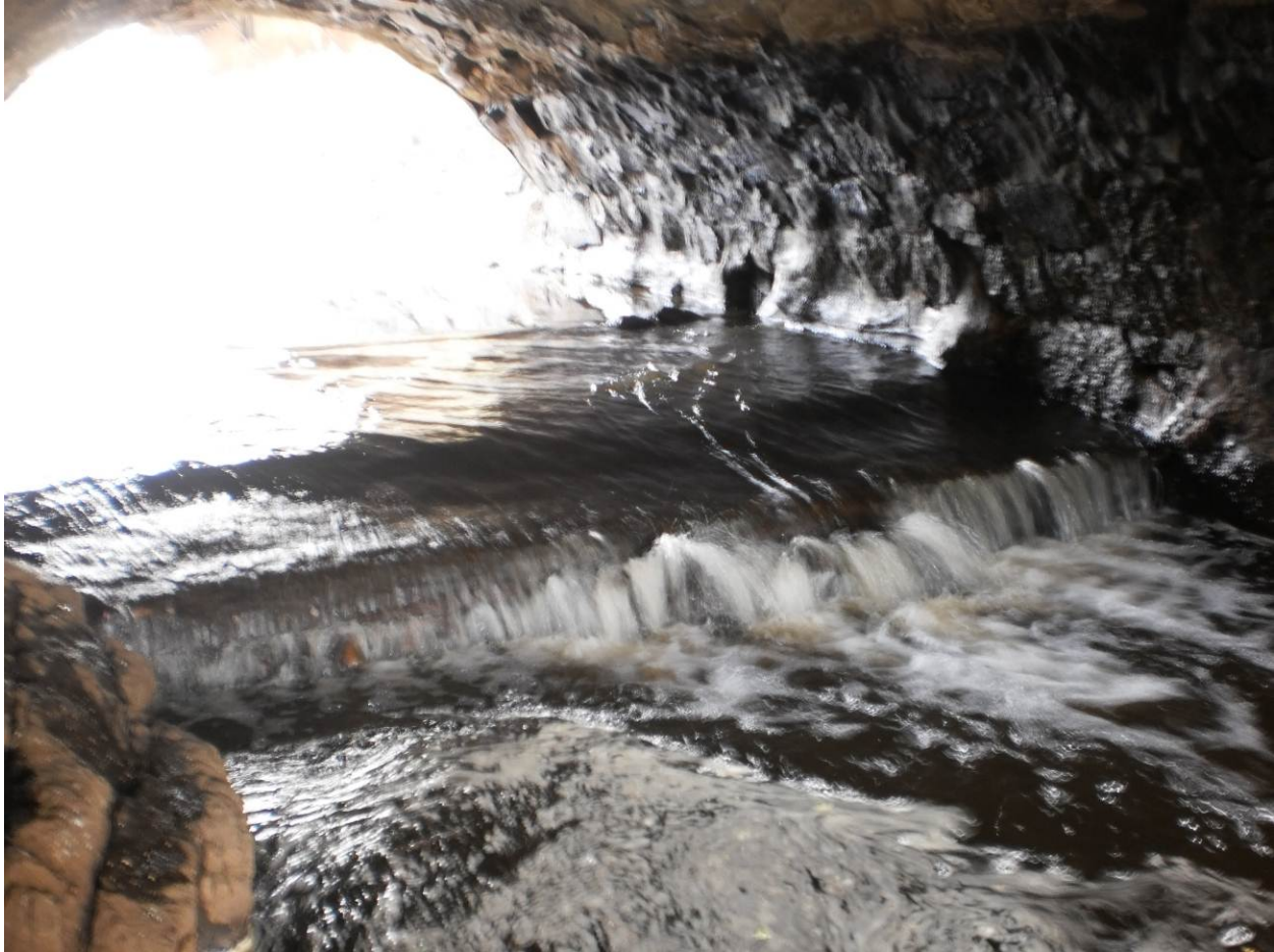
Photo 7 Mid length weir inside culvert, bedrock left
