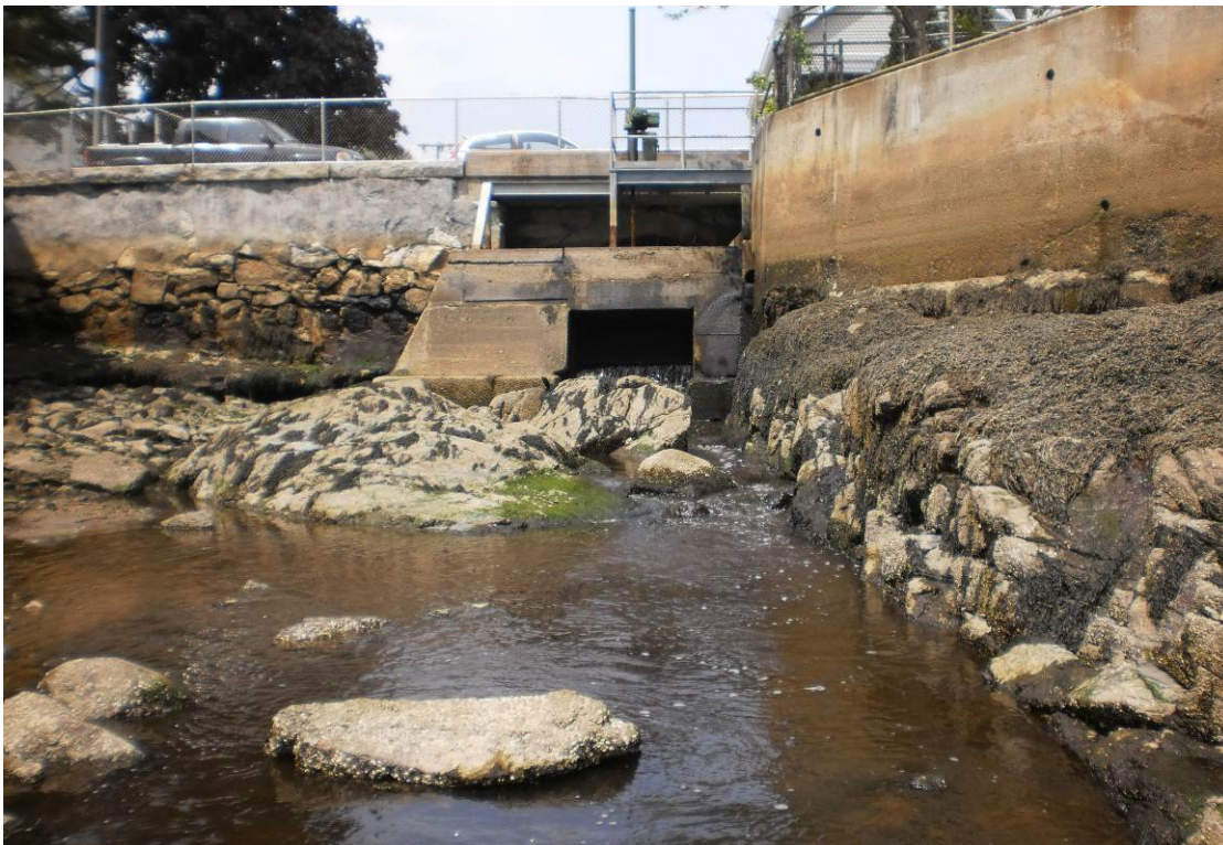
Photo 1 Looking upstream (low tide) toward tide gate and Central St culvert
