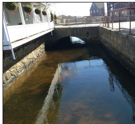
View of Central Street tide gate towards the Harbor
