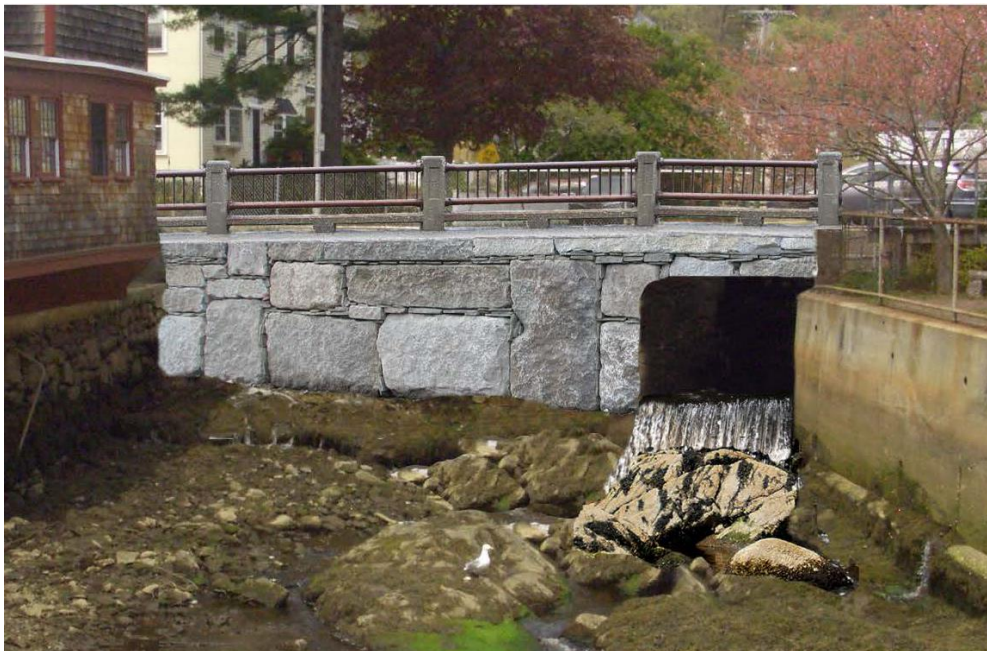
Figure 1 – Rendering of Granite Façade using Large Stones
