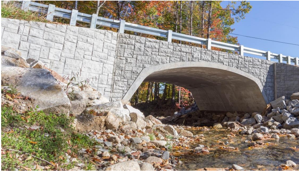
Figure 2 - Sample Concrete Formliner Appearance
