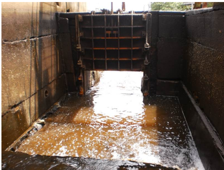
Photo 3 View of tide gate from inside culvert
