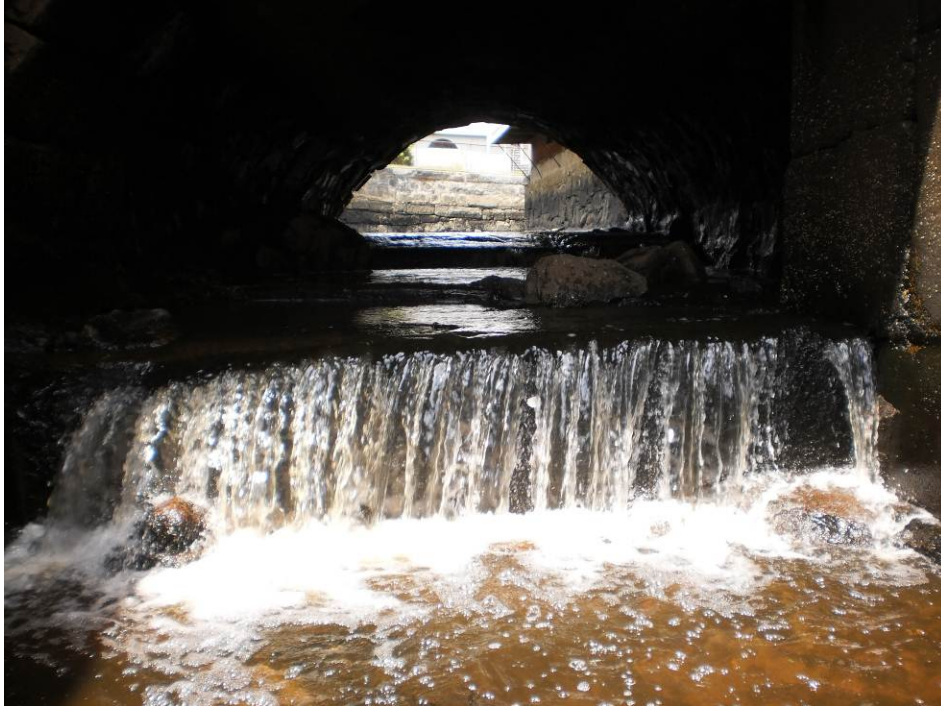
Photo 5 Downstream culvert weir looking upstream
