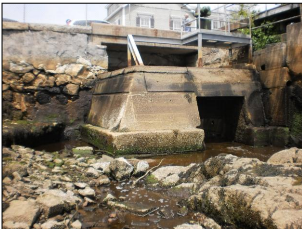
View of Tide Gate Structure from Harbor
