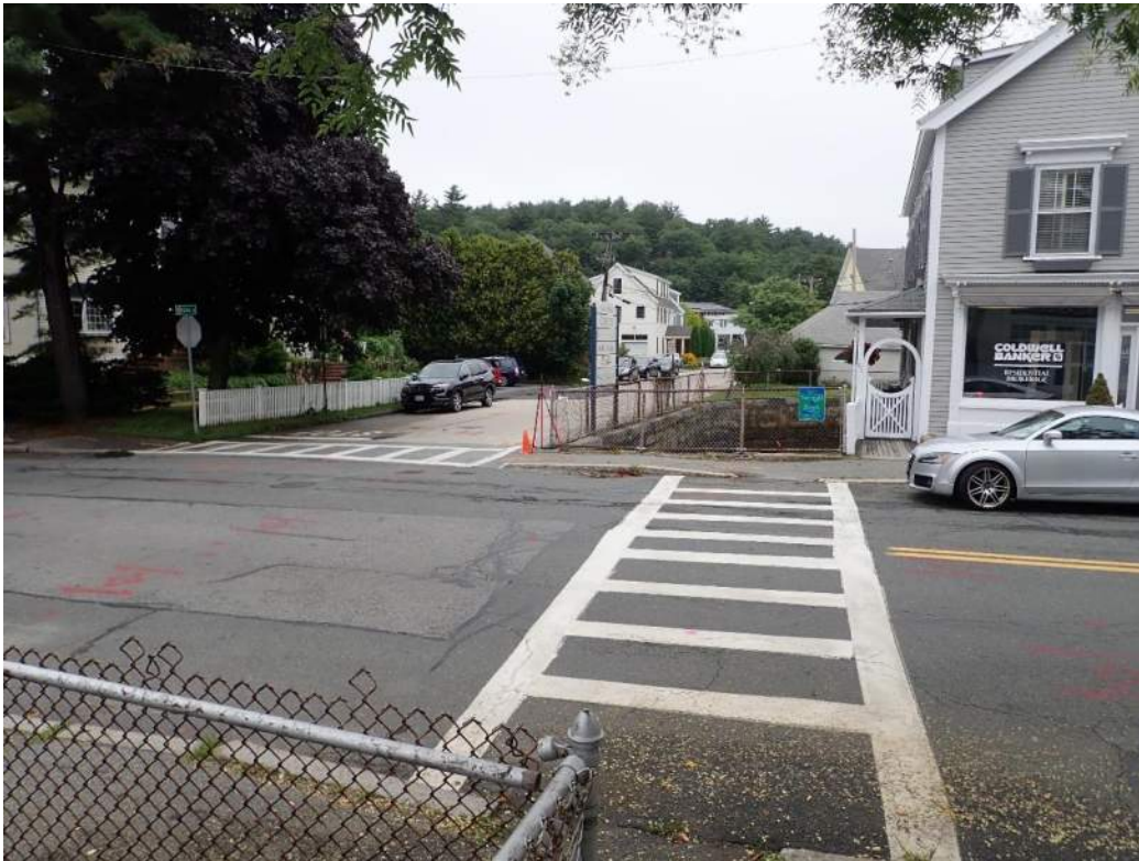
Photo 13: View of Central Street bridge, looking north / upstream toward Elm Street.
