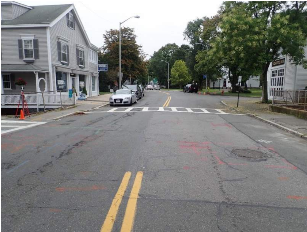
Photo 12: View of Central Street bridge, looking east (upstream is on the left side of the photo).
