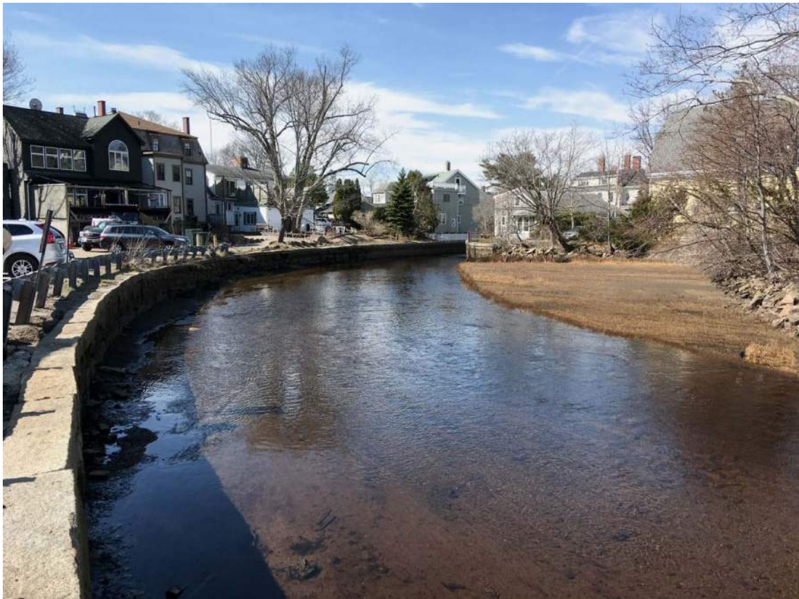
Photo 7 Before and After Restoration- South View
