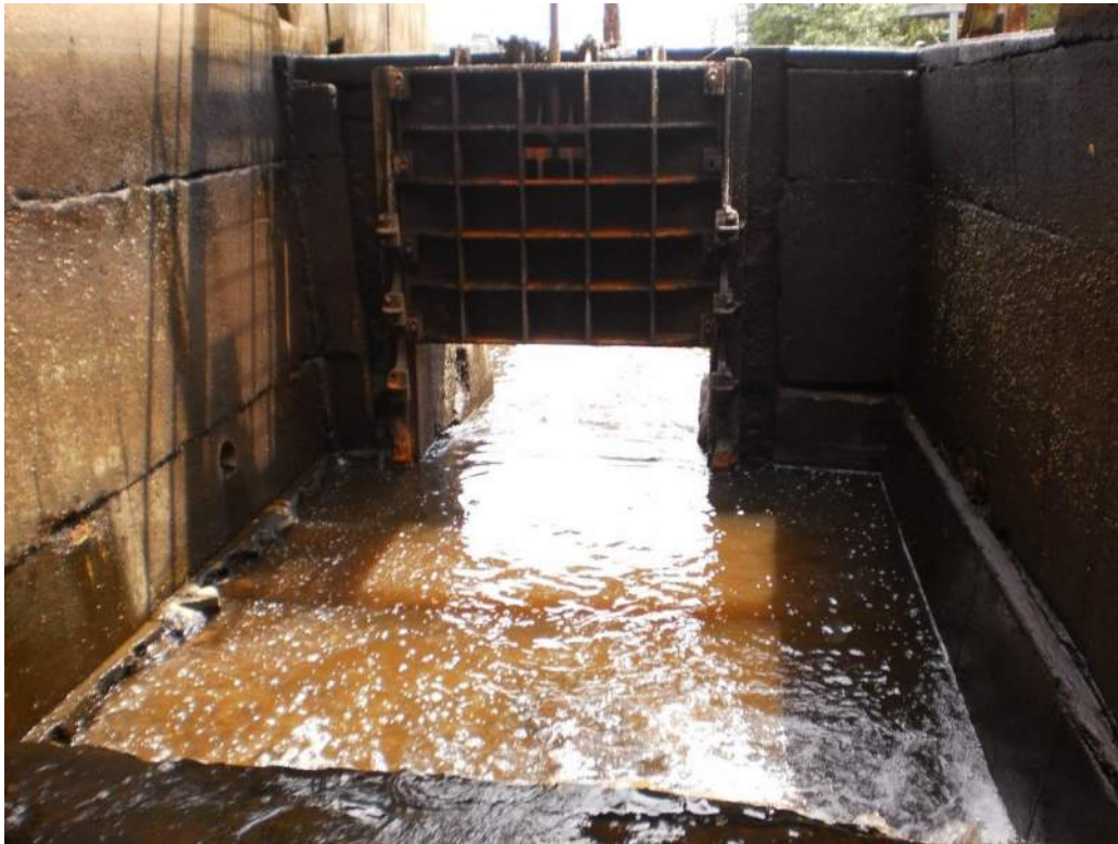
Photo 5: View of tide gate outlet from interior of tide gate chamber.
