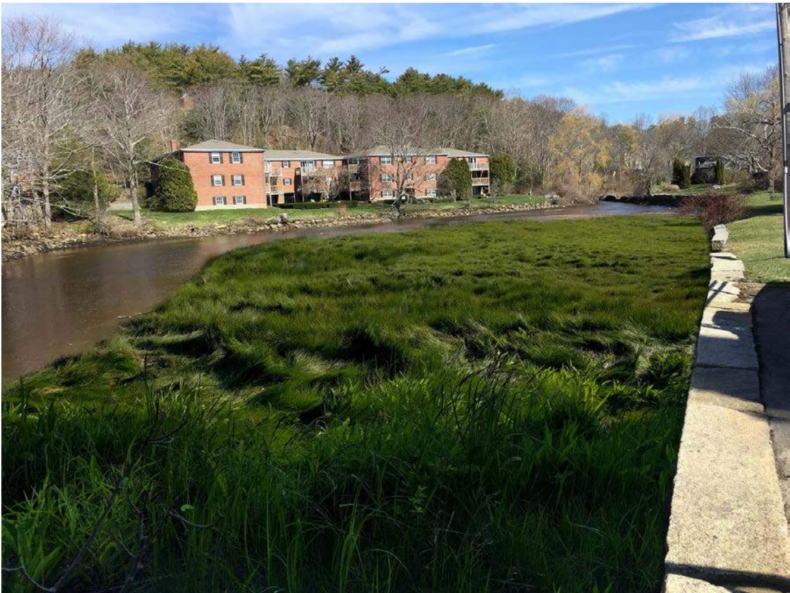
Photo 8 Before and After Restoration-North View
