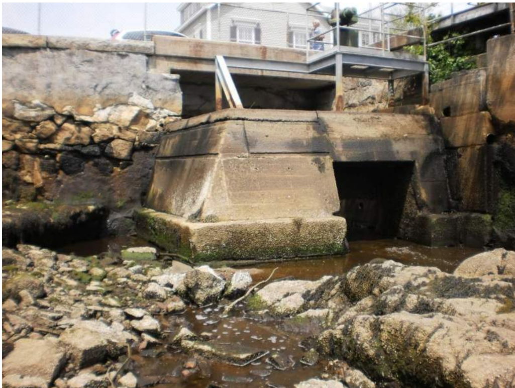
Photo 4: View of the existing tide gate from southwest.
