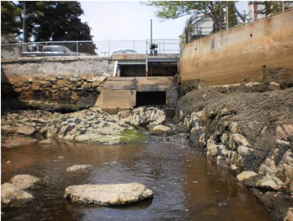
Photo 3: Central Street Bridge and tide gate from downstream.
