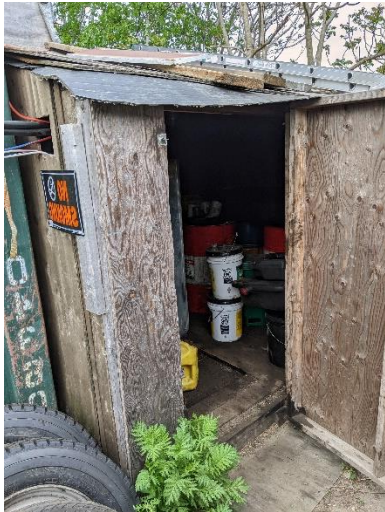
1. Containment shed w. roof
