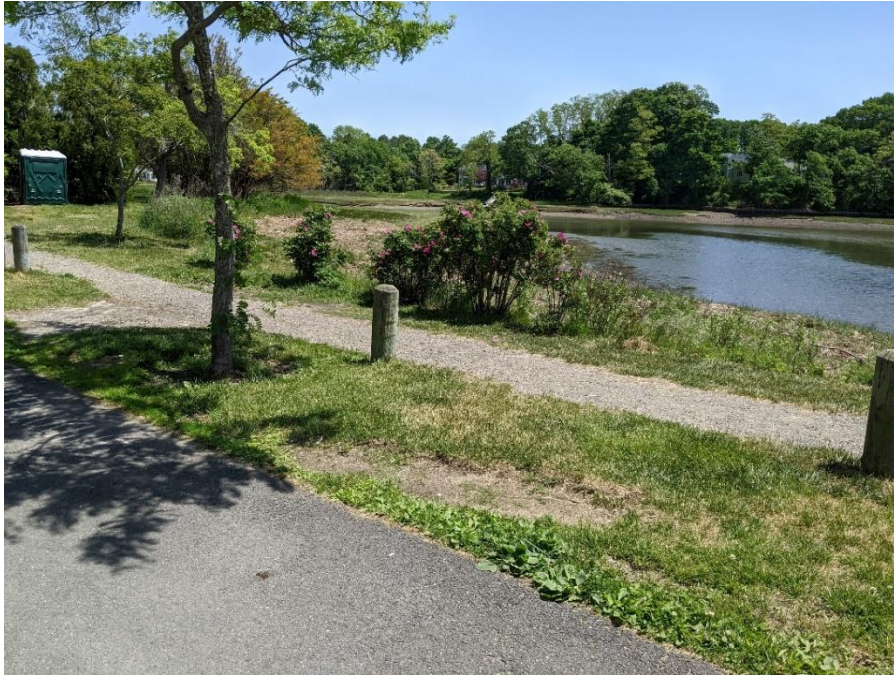
A more effective vegetated or stone filter strip could be used to slow water flowing from the parking lot into the marsh.
