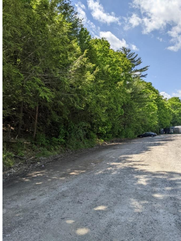
Bioswales could aid in water infiltration along the perimeter of the parking lot.
