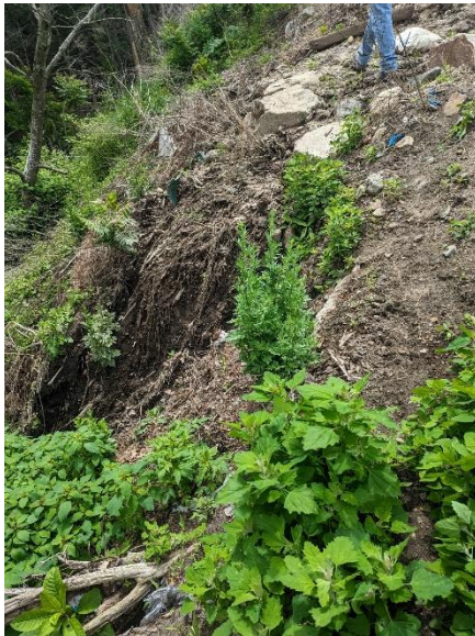
6. Erosion of slope
