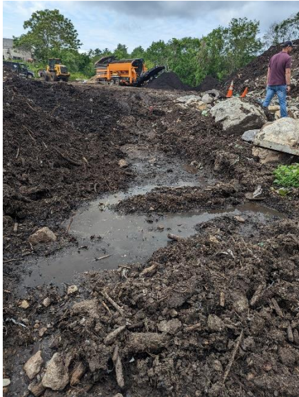
10. Pooling next to underdrain
