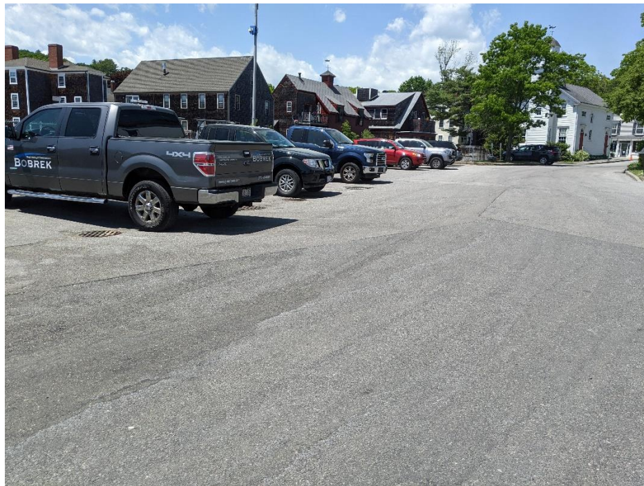
Five catch basins act as a pretreatment system for municipal vehicle washing station.
