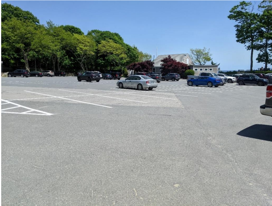
The Singing Beach parking lot could be retrofitted with vegetated islands and permeable paving to reduce the amount of impermeable land cover.
