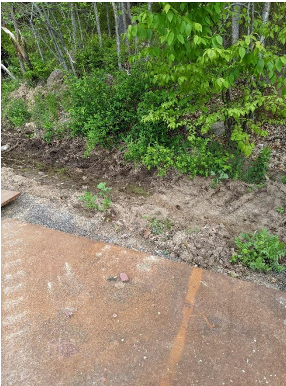
3. Swale Around Salt Barn
