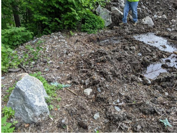
5. Pooled water next to steep slope
