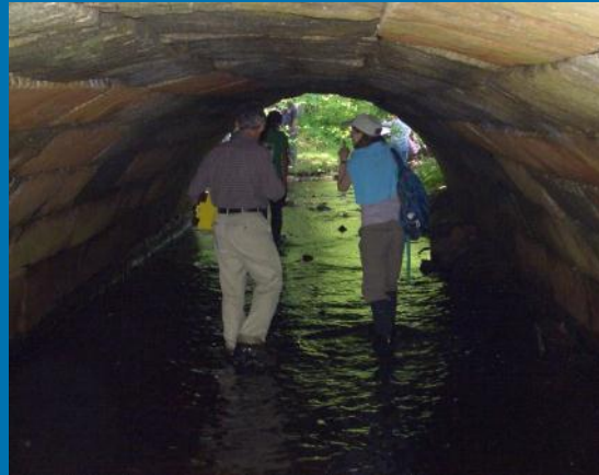
Assess adequacy of culvert sizes
