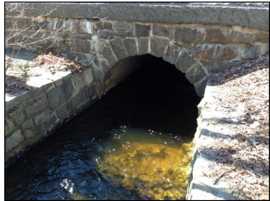
Inlet of School Street Culvert
