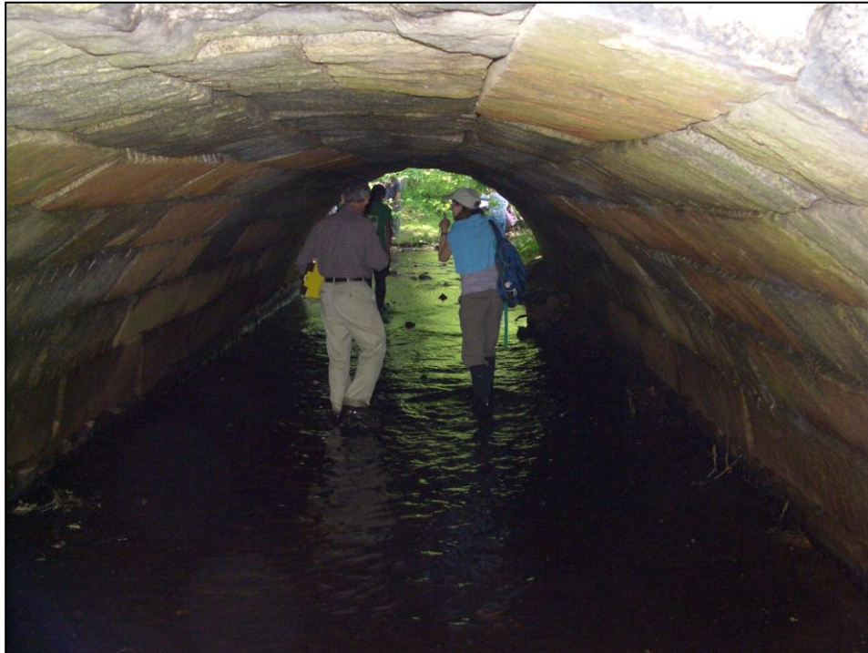
Stone Arch Construction of the Lincoln Street Culvert
