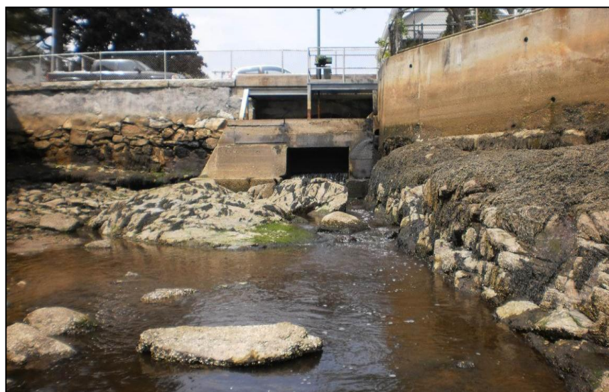
Looking upstream (low tide) toward tide gate and Central St culvert
