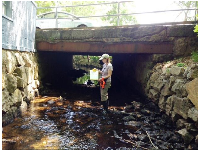
Outlet of Norwood Avenue Culvert
