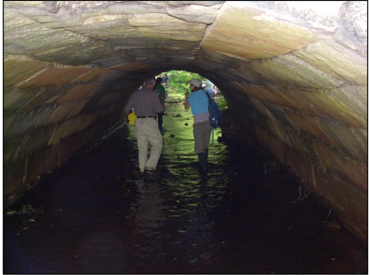
Town Staff and Volunteers making observations at the Lincoln Street Culvert
