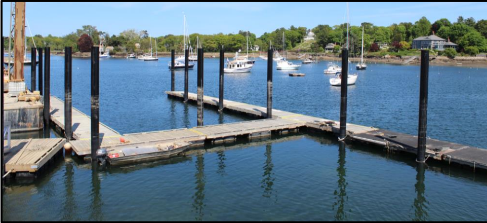
Rock Socketed Piles previously Installed at the Site
