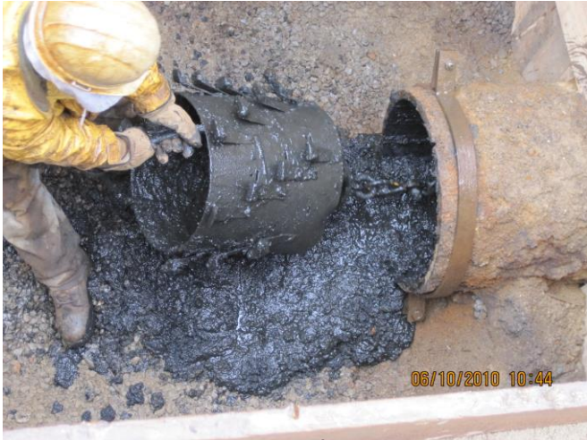
Water Main Cleaning
