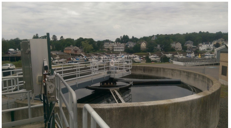
View of Manchester Harbor from the walkway above process equipment
