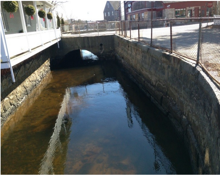
View from the south.
