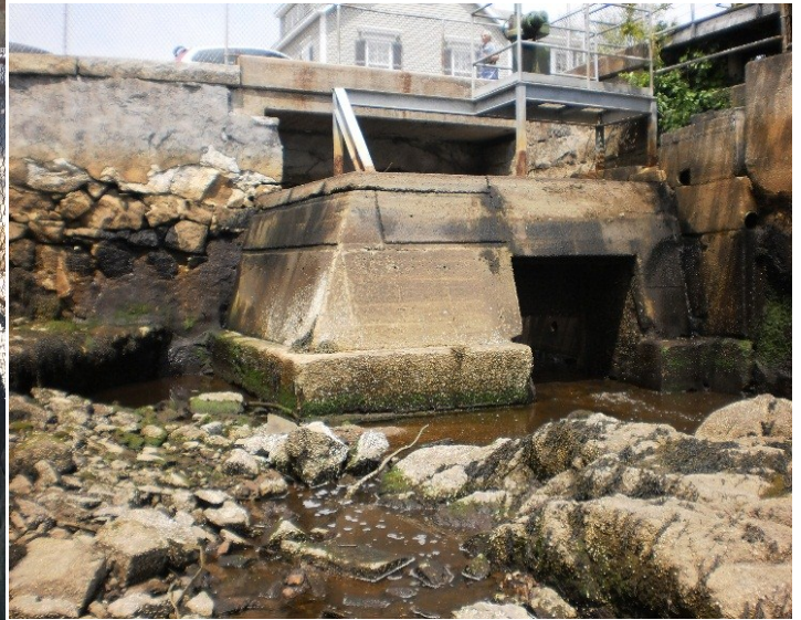
Existing tide gate.
