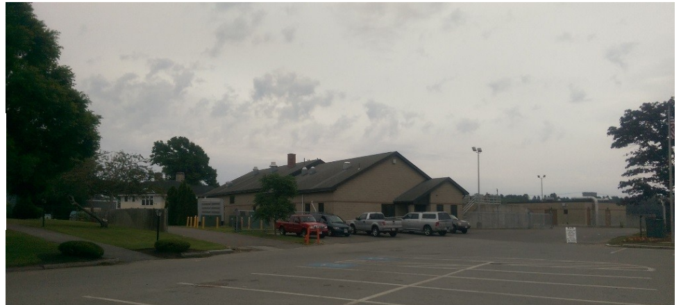
Manchester-by-the-Sea Wastewater Treatment Plant
